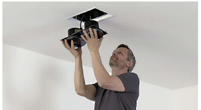
Connect the speaker module. Insert terminal into correct input on the integrated crossover.
