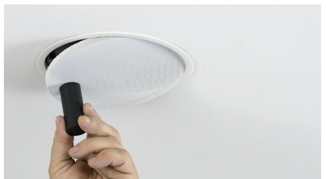
To adjust, remove the grille with the magnetic DE tool.
