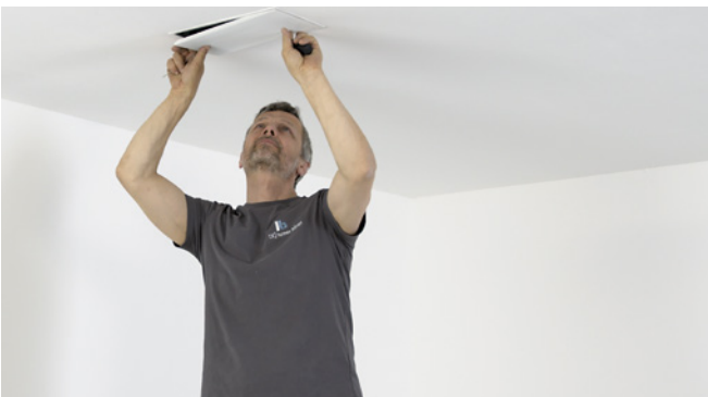
Insert the grille. Realign the fixing magnets if necessary. Revision: Remove the grille using the magnetic DE tool.
