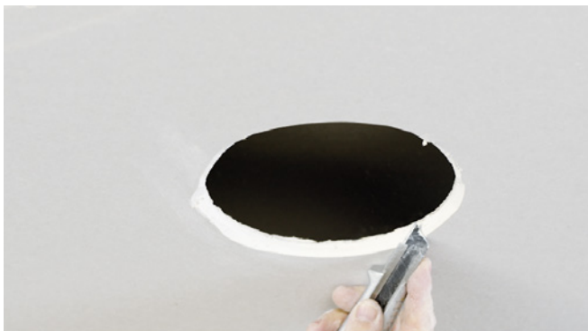
Trim the installation opening...
