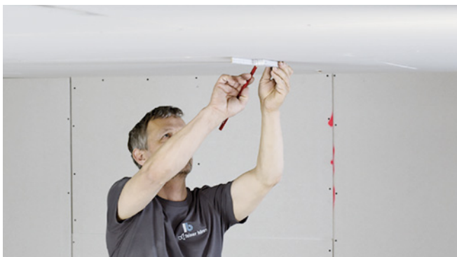
Locate and mark out the installation position.
