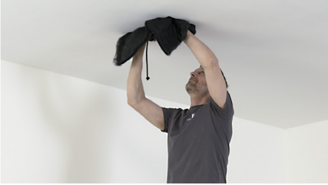
Line the box with insulating wool.
