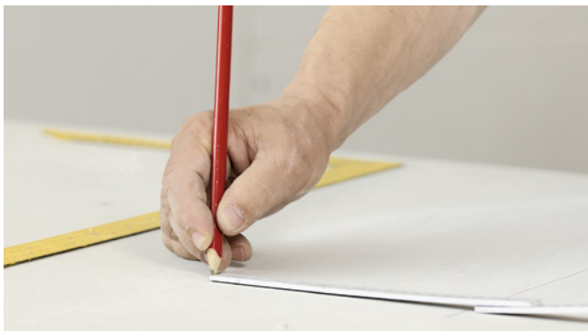
Locate and mark out the installation position.
