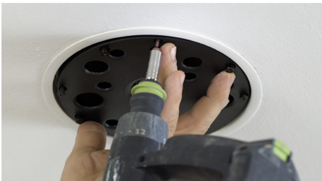
and fix in place.
