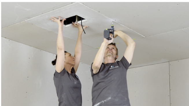
and screw the plasterboard in place.
