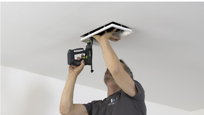
Insert frame into opening and screw in place. The springs are not used.
