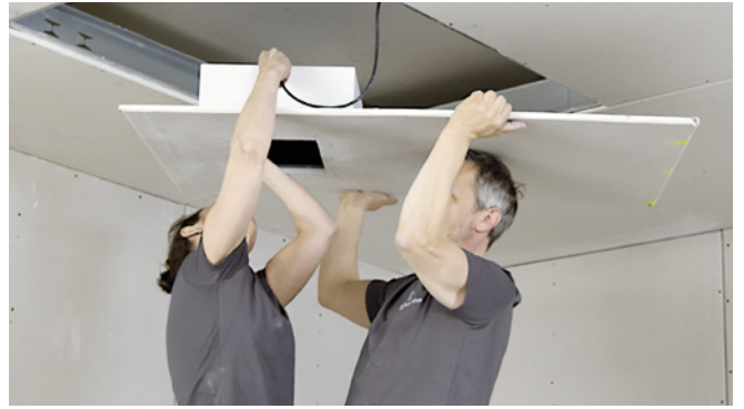
Guide the cable into the back box...
