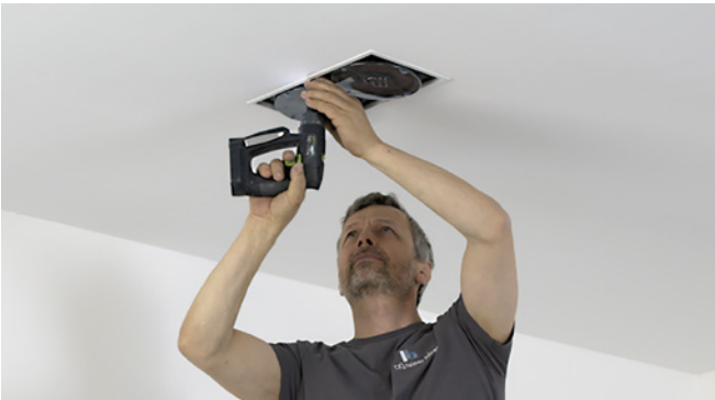
Insert speaker module and fix in place.
